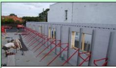
Walls braced and ready for placement of concrete. We can advise the most appropriate bracing approach for your project.
