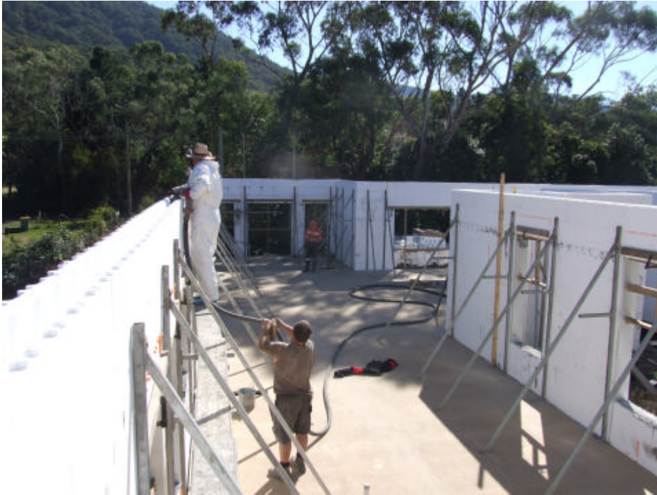
Note Lintelbricks clamped on the right of picture
