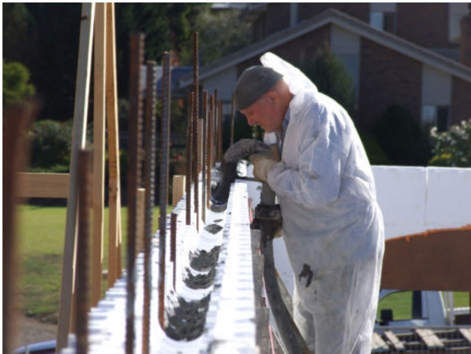
Concrete Pump with goose neck connection
