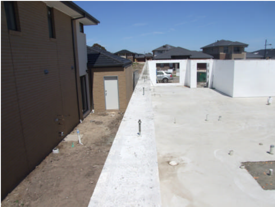
Bolts installed in readiness for top pitching plate to be placed
