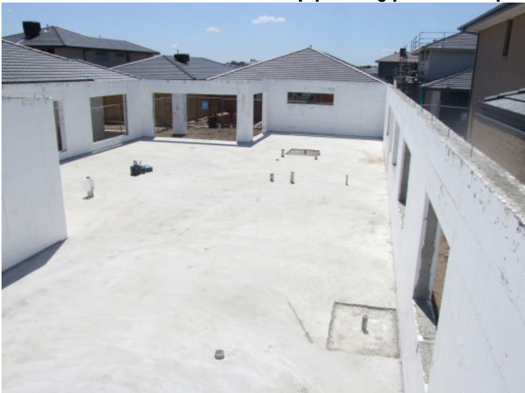
Bracing stripped and project is ready for framing
